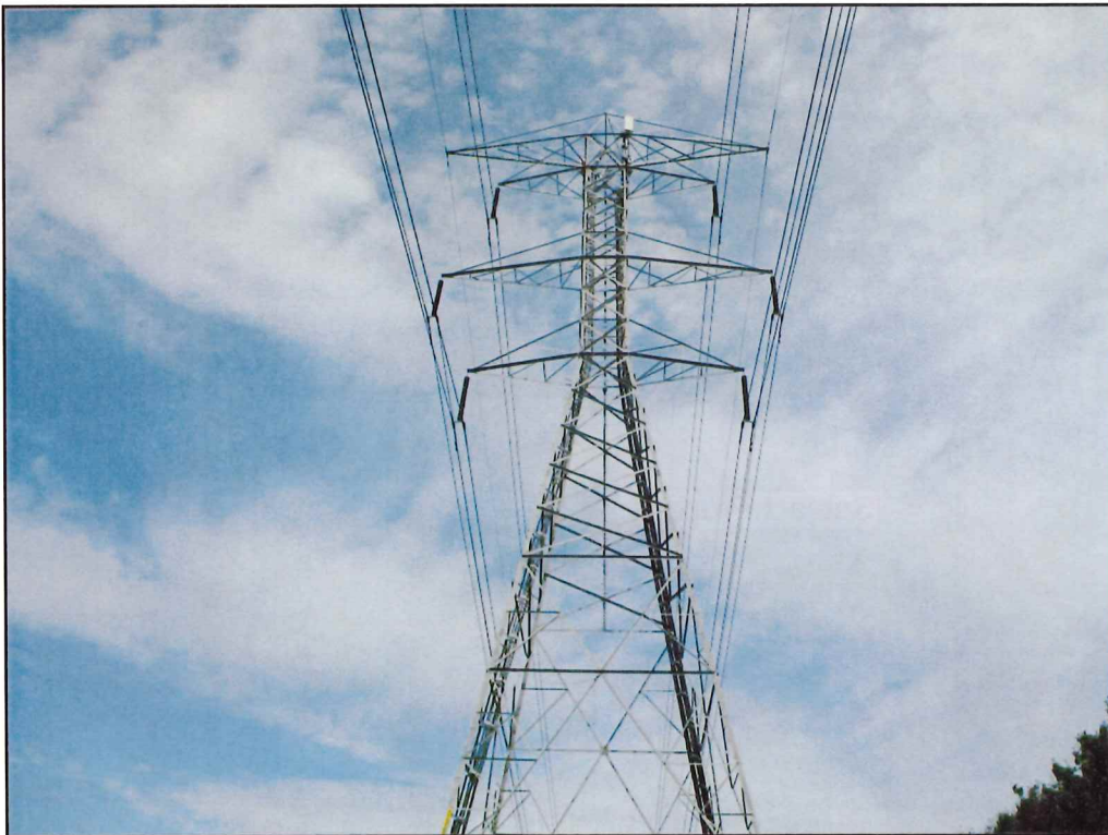
Photograph 2 – Subject property, facing east.
